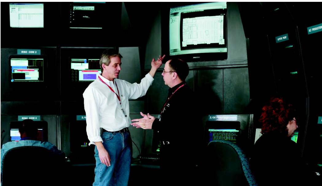
Matt Phillips (left) of TECH SITE with Safelite’s Randy Randolph in the Safelite network operations center. Through SiteScan Web, Safelite can continuously monitor critical support systems across three facilities from the operations center.
