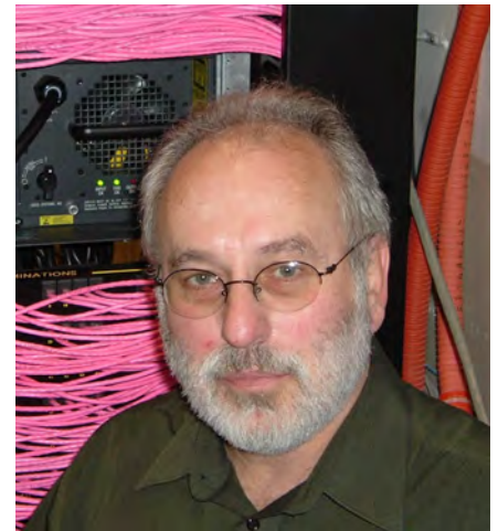
Ron Kasper of Marquette University with one of the school’s IP telephony installations.
